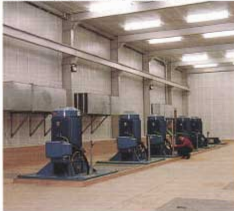
Water Pumping Station, Egham, England
